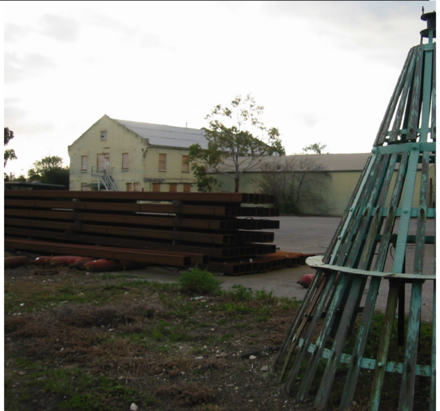
The Dockyards with the brick Riggers and Transport offices in the background, Aug 2003
