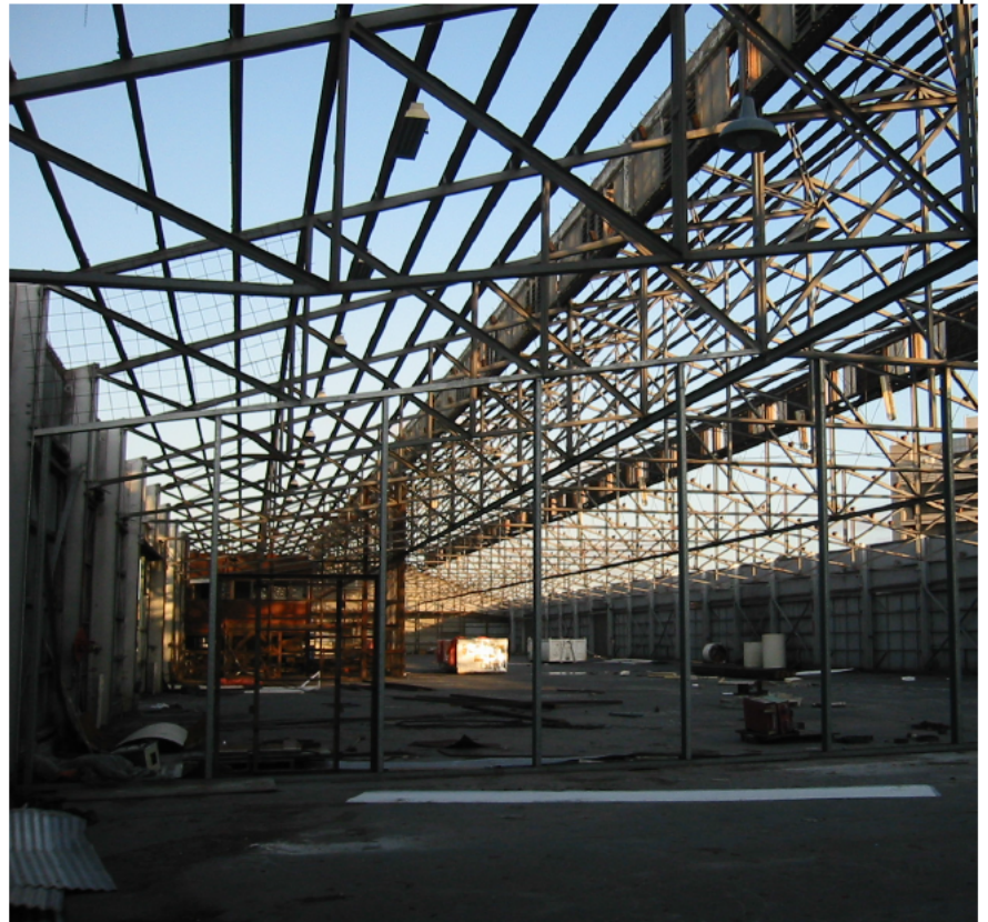
Shed #5, asbestos roof removed, about to be demolished
