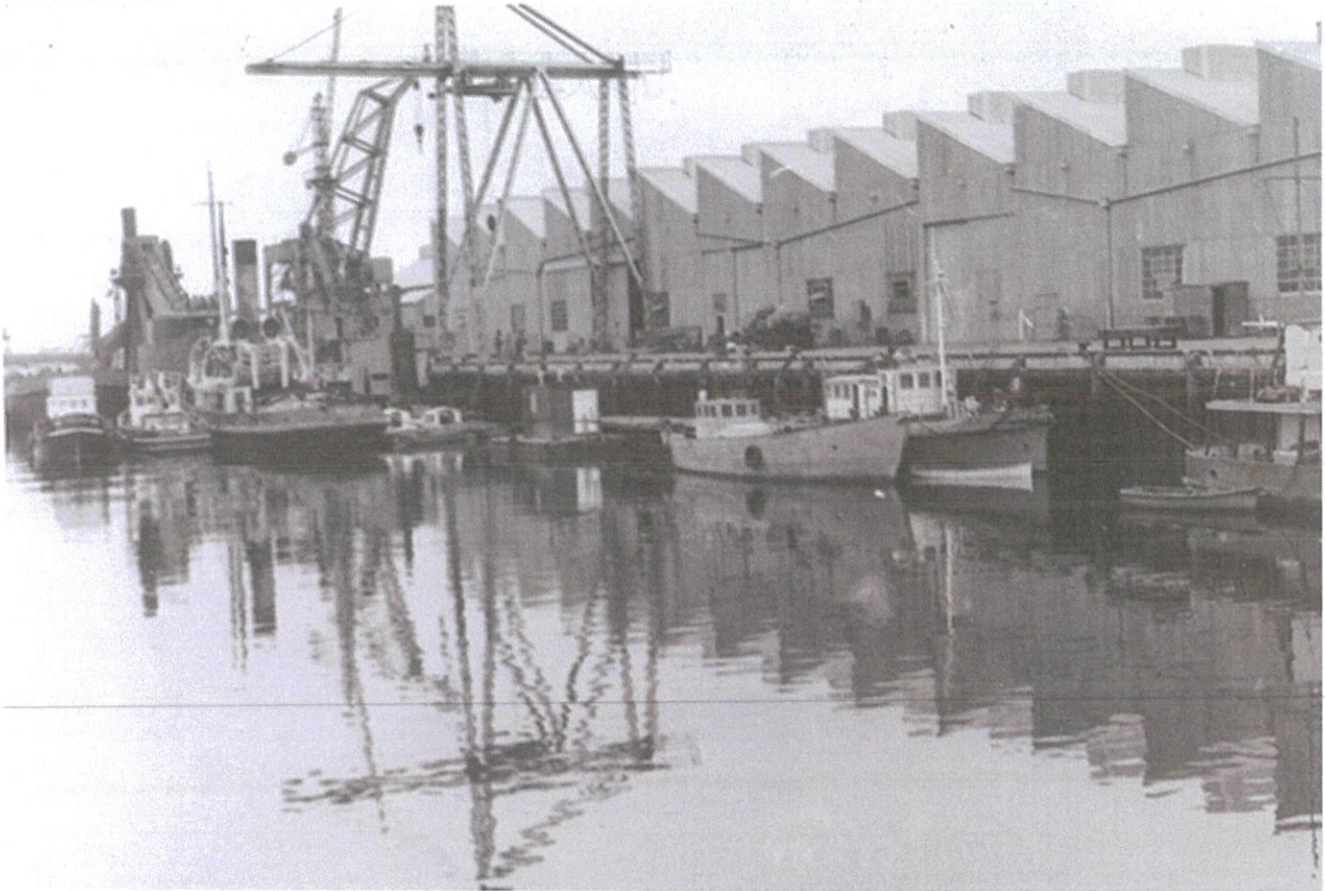
Glanville Dockyard with dredges and mooring vessels SA Maritime Museum Collection
